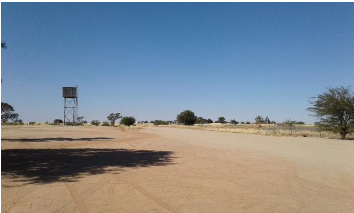
Figure 5: Water tank at Grünau
